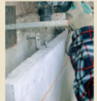
stone being lifted into place on wall
