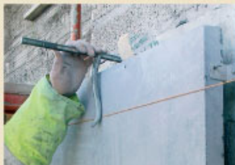
temporary clamp to hold stone in position
