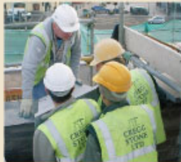
stone being lifted into position for measuring and boring
