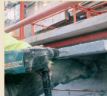
boring of holes for fittings
