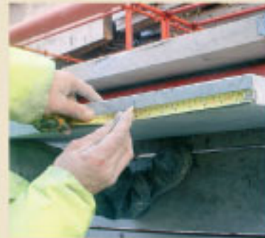
measurements being taken for holes
