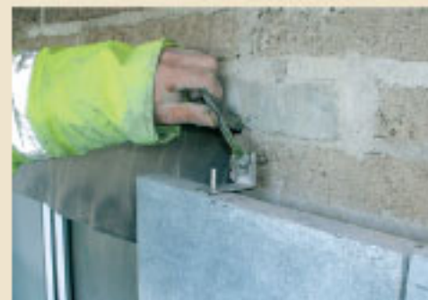
retention fixing plus dowel to secure stone to wall
